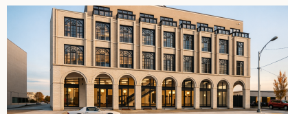
WEST FAÇADE ALONG NW DAVIS ST.
