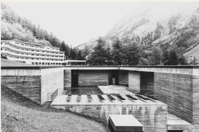
Figure 5 – Peter Zumthor, Therme Vals, exterior view
